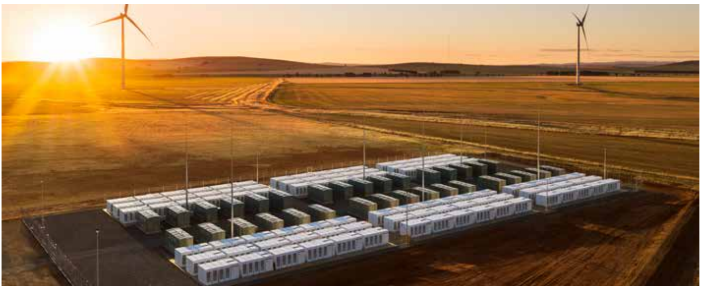
Figure 43: Hornsdale Power Reserve in South Australia
