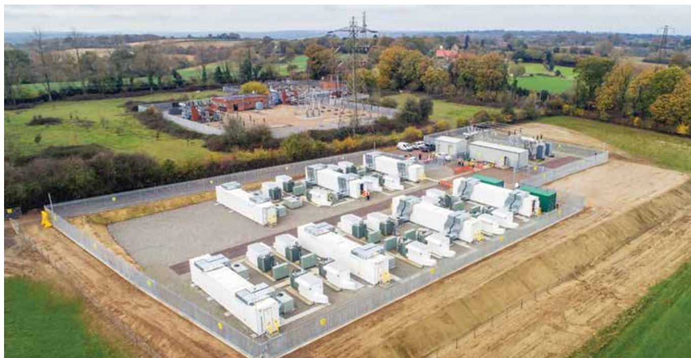
Figure 31: Low Carbon’s Glassenbury project
