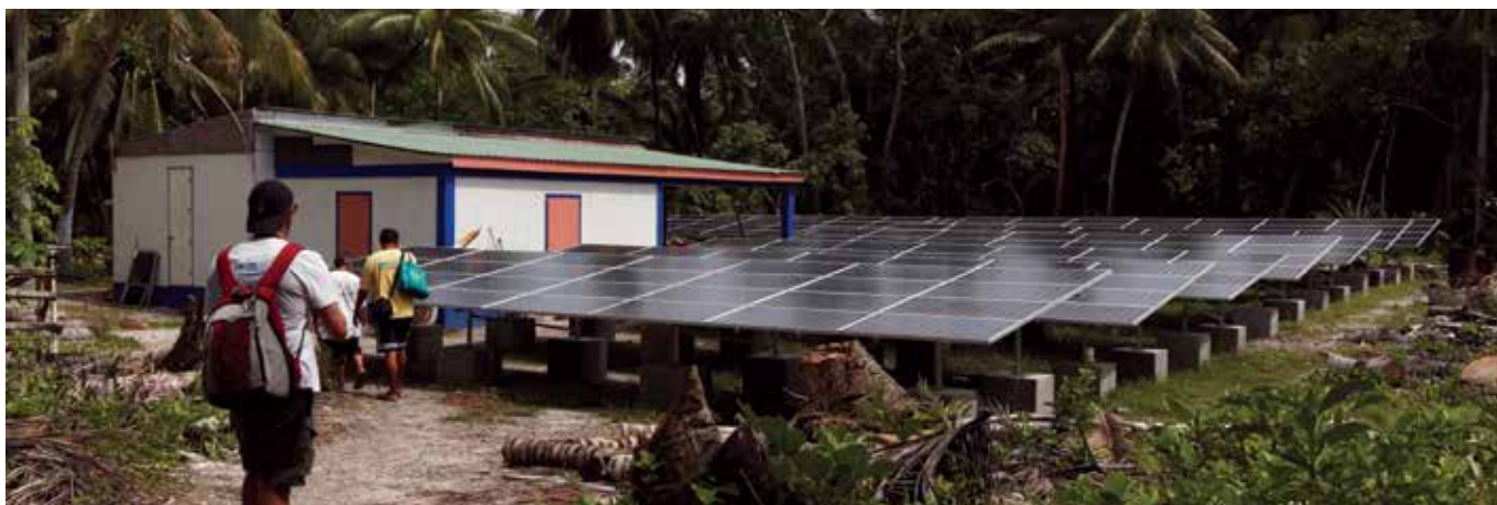
Figure 59: Inspection of a solar mini grid in Mog Mog, Ulithi atoll, Yap State, FSM
