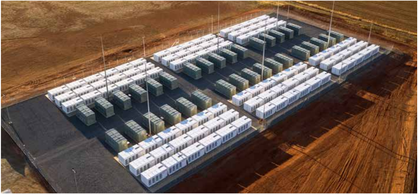
Figure 32: Hornsdale power reserve project in South Australia
